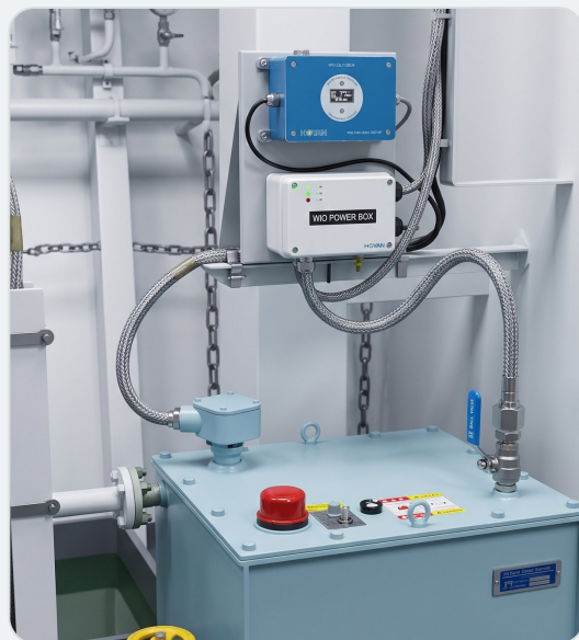
WIO-23LY-DBOX + POWER BOX · in-situ tank installation
